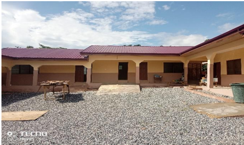
Completed 2no. 6unit Classroom Block with Office & Library at Nyame Nti & Suponso
