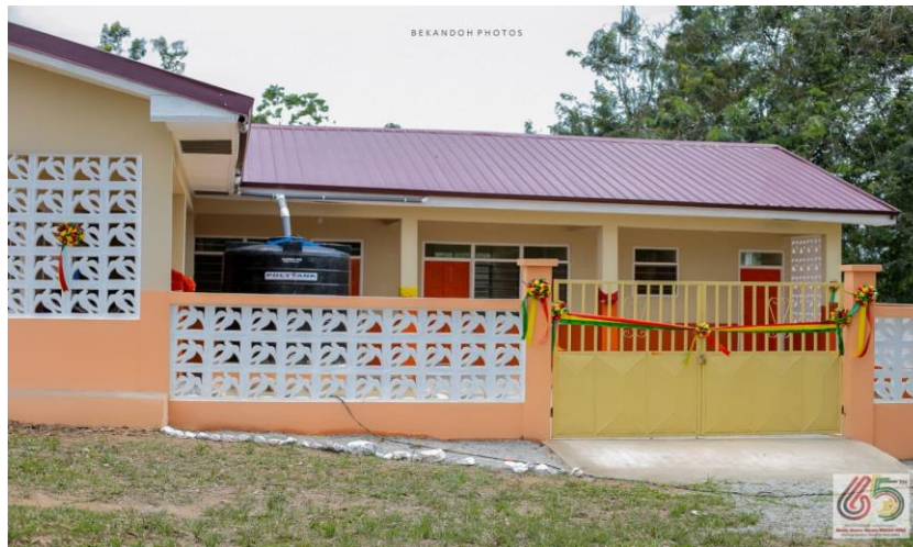
Completed 1no. KG Block at Manso Presby
